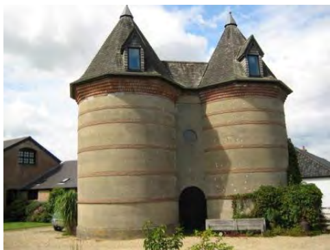
13. Silos designed by Max, Briantspuddle, Dorset.
