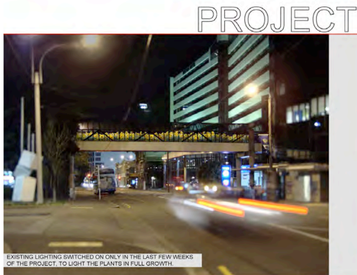
Fig. 7: Project: Street view of bridge with intervention at night
