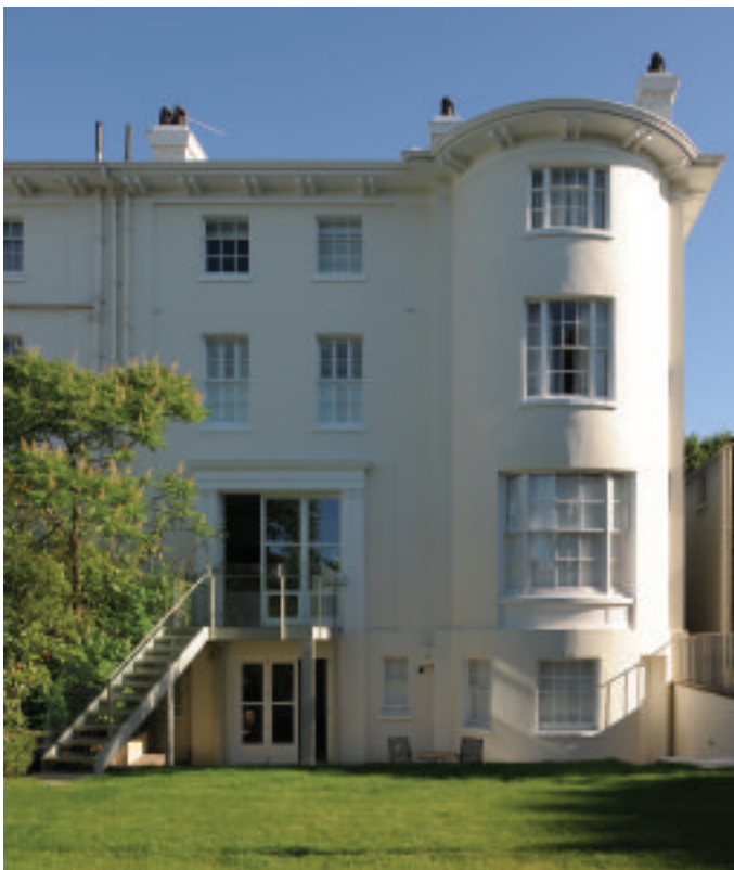
Rear of house with balcony and staircase
