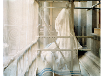
Photograph by Mark Power - refurbishment of The Treasury in London
