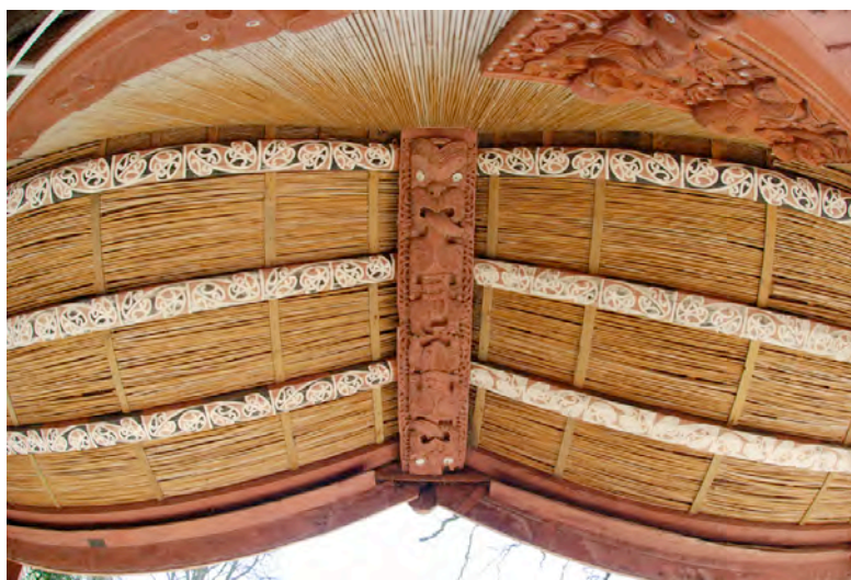
Image 3. The carved, painted and tied panelling of Hinemihi’s porch. Photography by the author.
