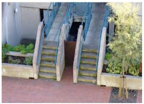
**Fig. 3:** View of parallel stair and bridges leading to lower maisonettes, block B. Note the blocked off entry to the lower level between the stair.
