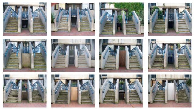
**Figs. 7-18:** Examples of modifications to the passageway leading to the lower level of the maisonettes in block B. The first is an example of an unmodified passage.
