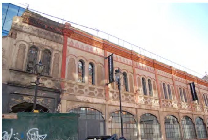
Figure 2. This photograph of the Moorish Market Hall, taken in February 2009, shows the ornate façade. The building was under refurbishment at this time, with a contemporary glass insertion constructed in place of the fire-damaged structure.
